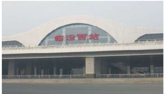
Shanxi Linfen High Speed Rail Station
